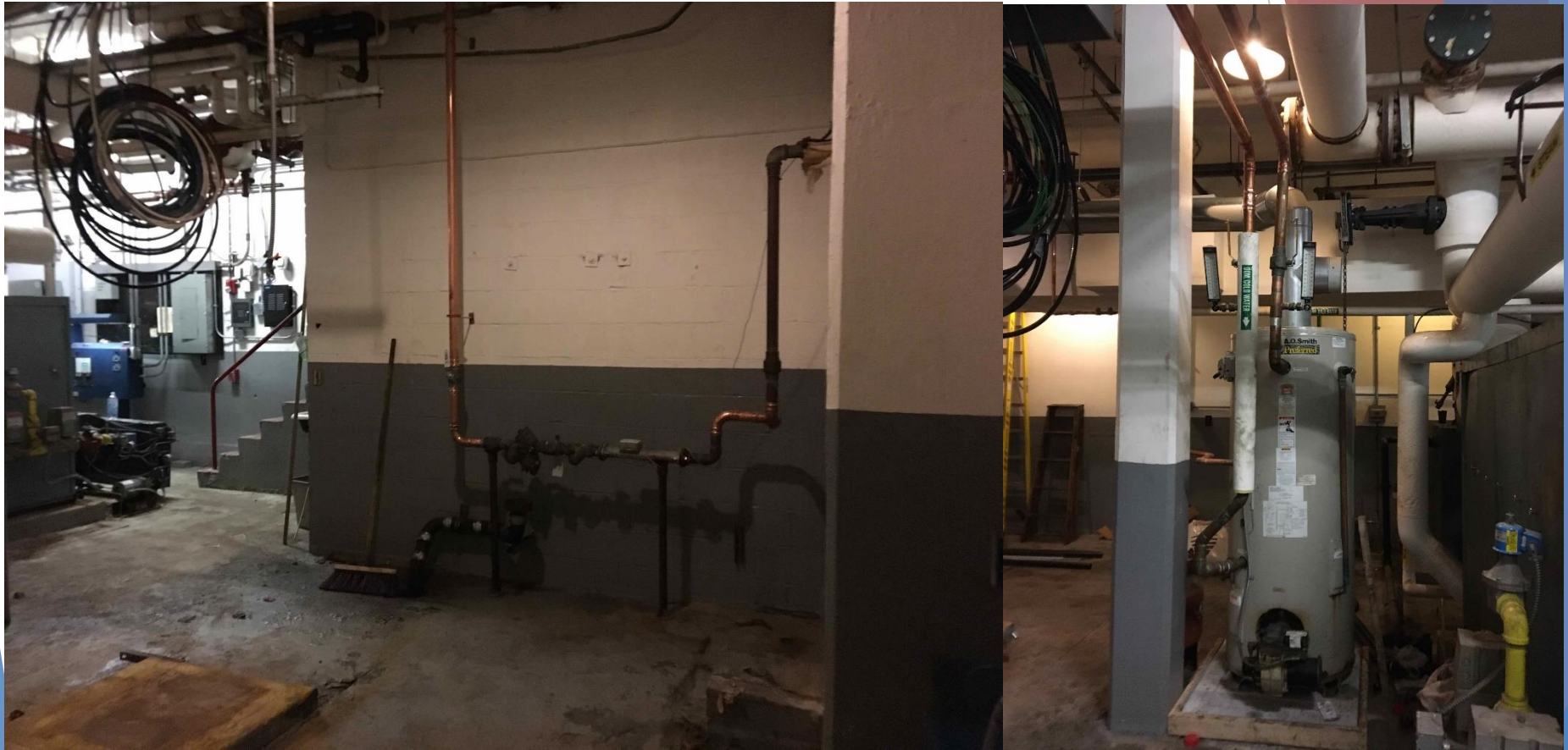
Relocated water main and hot water heater.
